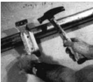
1 Tap shoulder rivets on mounting brackets into slotted key-holes on the track.
