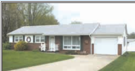
1101 NE 3RD STREET
