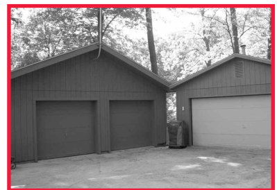
Two 2 car garages one with electric & water. Concrete driveway plus carport.
