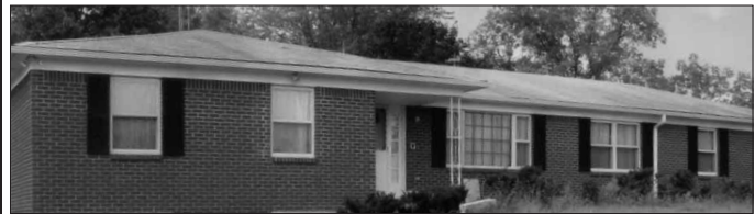
LOVELY BRICK HOME IN COUNTRY- 3 Bedroom, 3 bath, living room, dining room, large family room, full walkout basement, 2 fireplaces. 2 car garage, 30x60 storage shed. All on 5 Acres.
